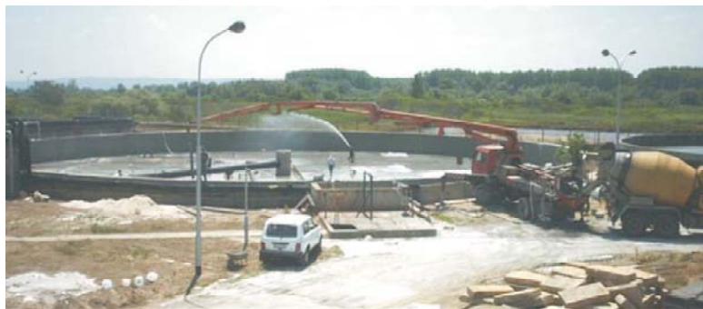
Trickling filter reconstruction
