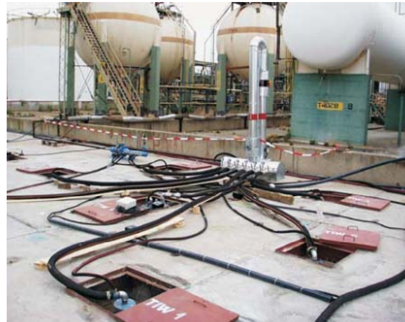
Groundwater remediation, pilot testing
